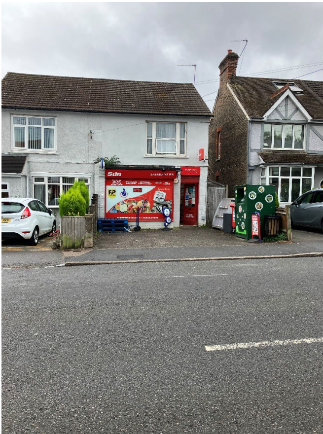
Views to the front of the store
